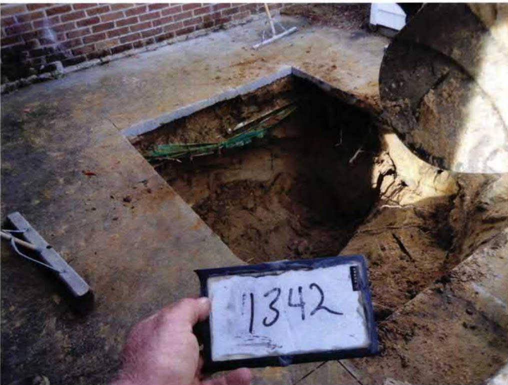
Picture 2: UST 1342Albatross excavation.
